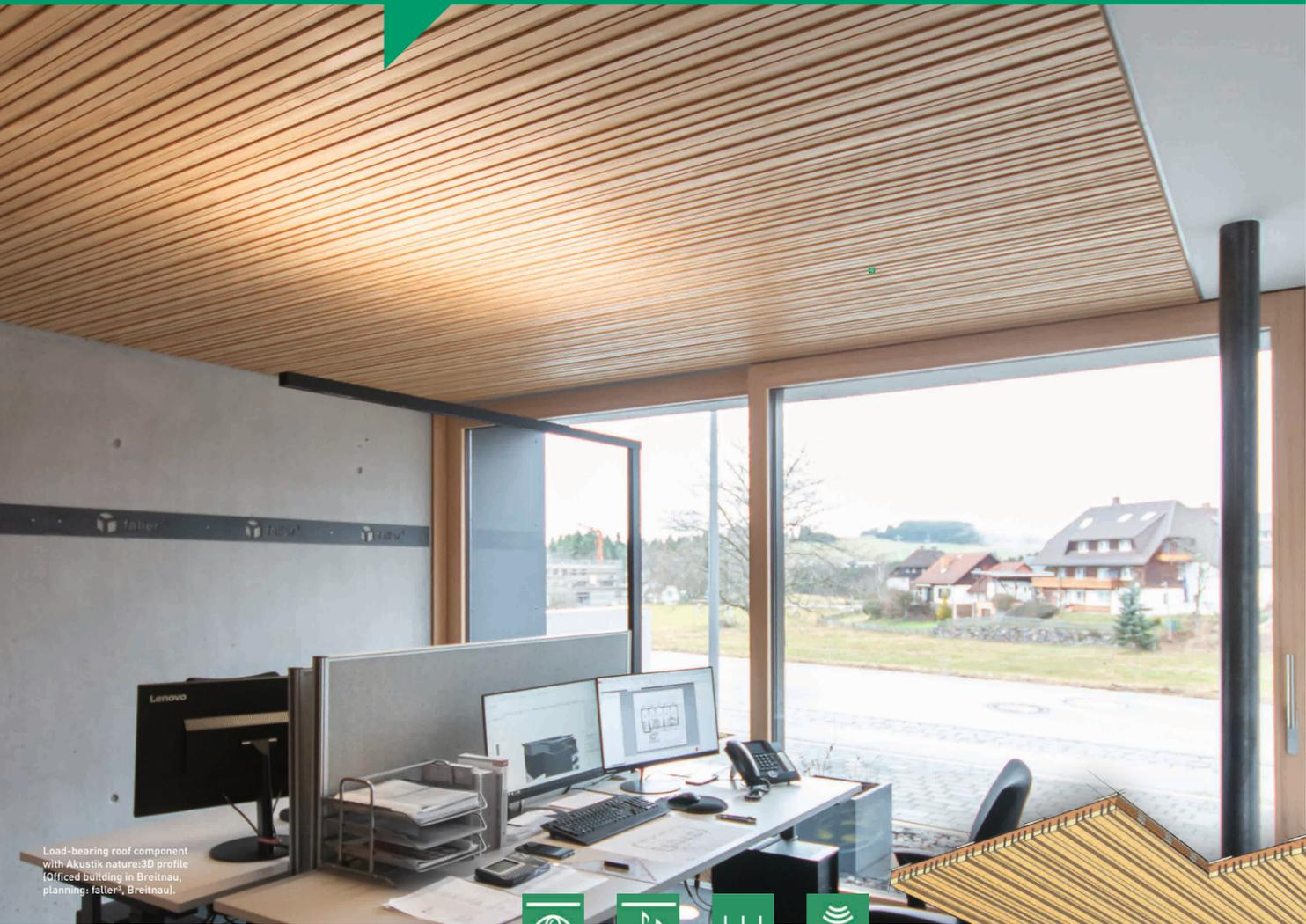
Load-bearing roof component with Akustik nature:3D profile (Officed building in Breitnau, planning: faller³, Breitnau).
