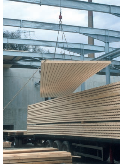
Preassembled large-area modules during installation
