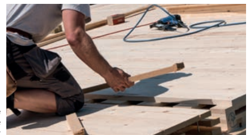
Insertion of the absorber strip in the lateral element joint
