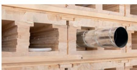
Ex works installation of ventilation ducts (spiral ducts) in BV elements
